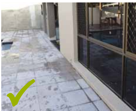
These windows have fixed security screens.
