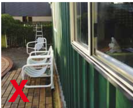
Windows that provide easy access to the pool area must be secured.
